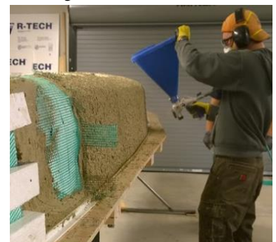
Figure 16: Shotcrete Spray Method
