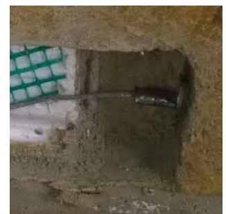
Figure 12: Button-Stop System
